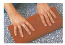
13. Trim off excess floor covering along the walls and skirting boards.
