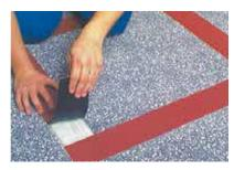
I. Using a rubbing board, press border firmly into place.
